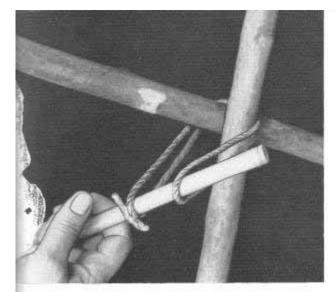
Strop and Turning Bar at start of operation.
