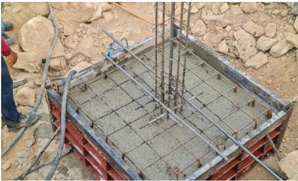
Concrete reinforced with steel bars (rebar)
