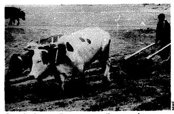
Fig.6 Ox-drawn soil scoop excavating a pond.
