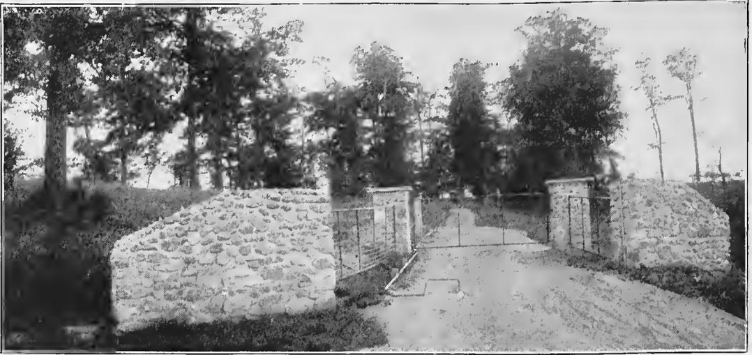
FIG. 250—STONE ANCHOR-WALLS FOR FENCE.
