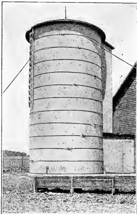
Fig. 294. A good stave silo well anchored.
