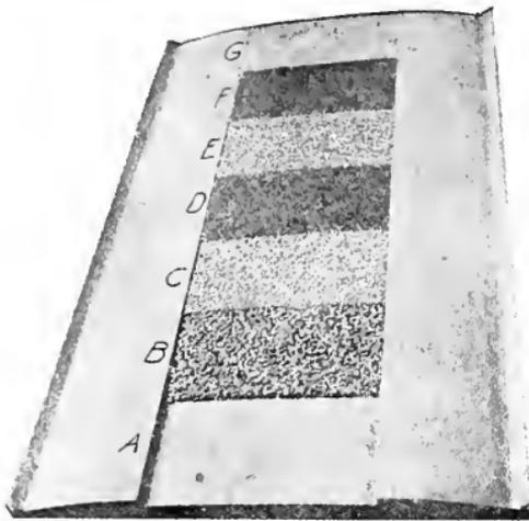
Fig. 86. Model of a bituminous macadam road made by the penetration method. *A* represents the prepared sub-grade. *B* represents the first course of stone, and *C* the second course. *D* shows the first application of bitumen. *E* shows the application of a course of stone chips. *F* shows second application of bitumen. *G* shows the completed road with a layer of clean stone chips, lightly rolled. (Bul. 36, Office of Public Roads, U. S. Dept. of Agr.)
