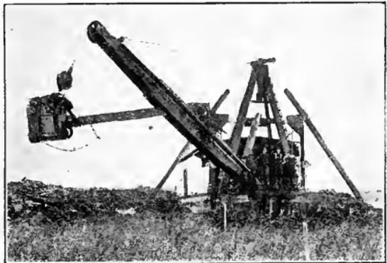
Fig. 65. A floating dredge for digging open ditches.
