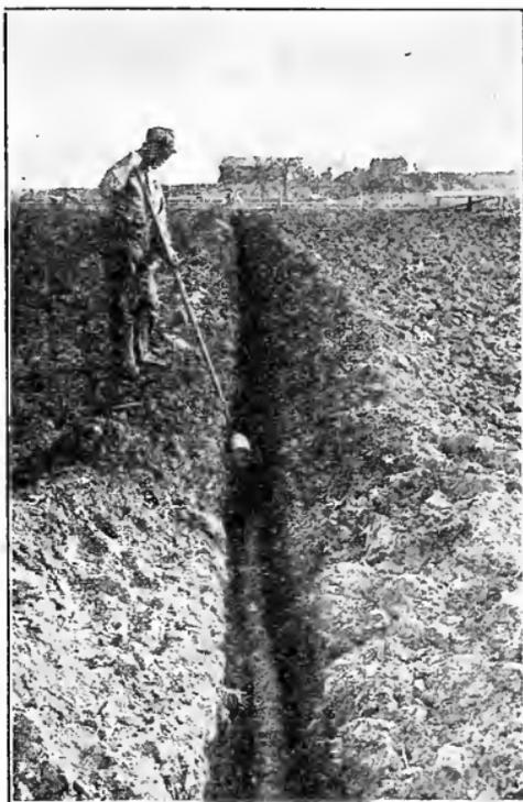
Fig. 59. Laying tile with the tile hook.
