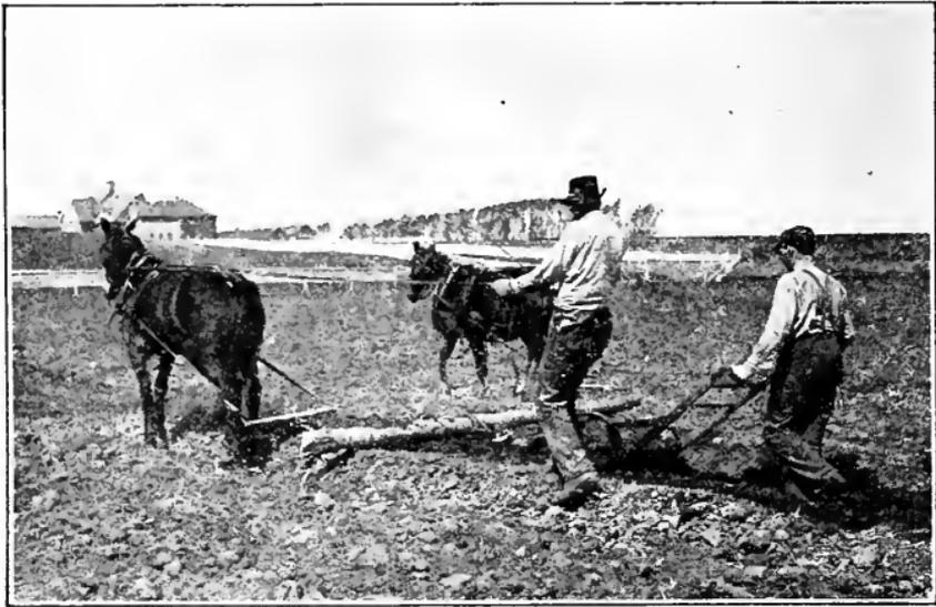
Fig. 61. Filling the ditch with a plow.
