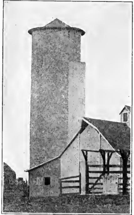
Fig. 304. An Iowa silo with a masonry water supply tank on top.
