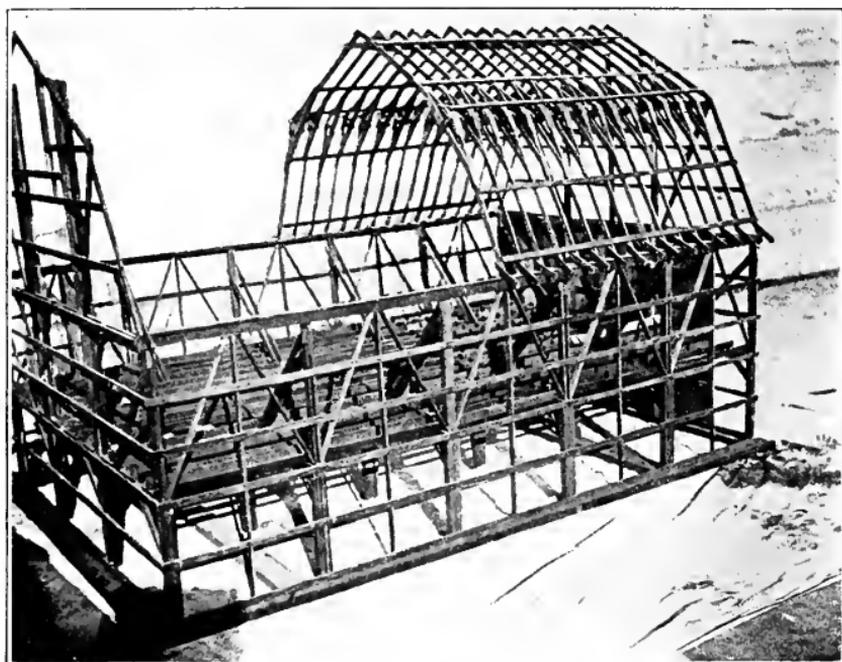
Fig. 287. A model Wing joist barn frame.
