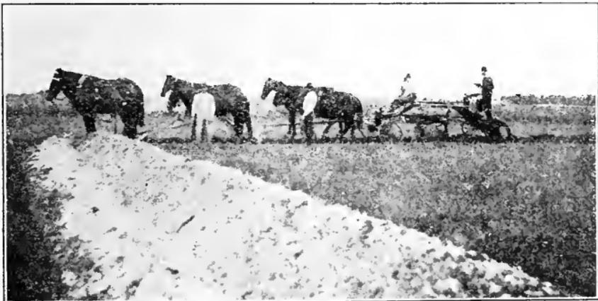
Fig. 62. Filling the ditch with a road grader.
