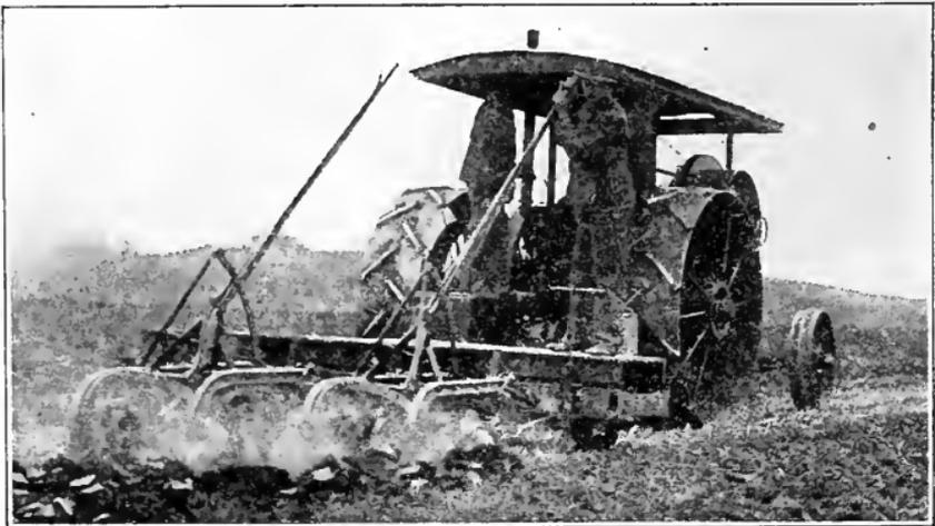
Fig. 236. A small gas tractor plowing. It may be successfully operated by one man.
