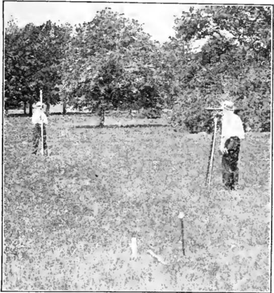
Fig. 50. Taking levels in making a survey.
