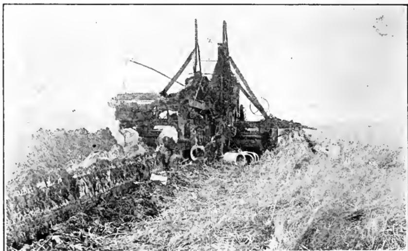
Fig. 55. A large tile ditching machine at work.
