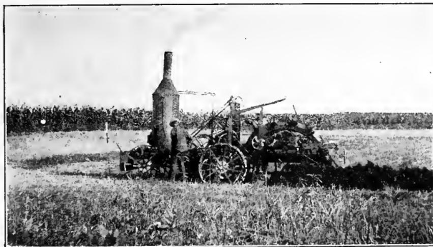
Fig. 54. A tile ditching machine at work.
