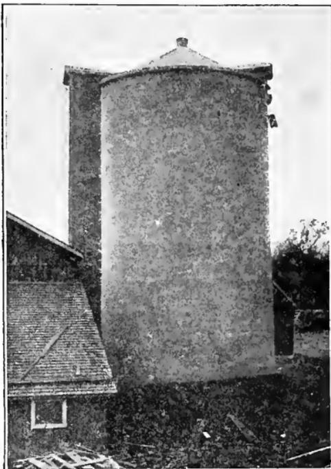
Fig. 295. A monolithic silo with concrete roof.
